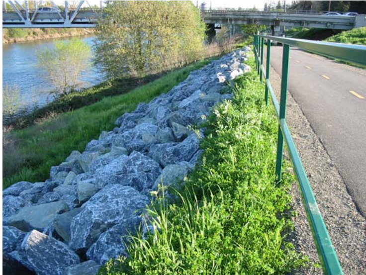
Figure 29 – Rock/Boulder Retaining Wall
