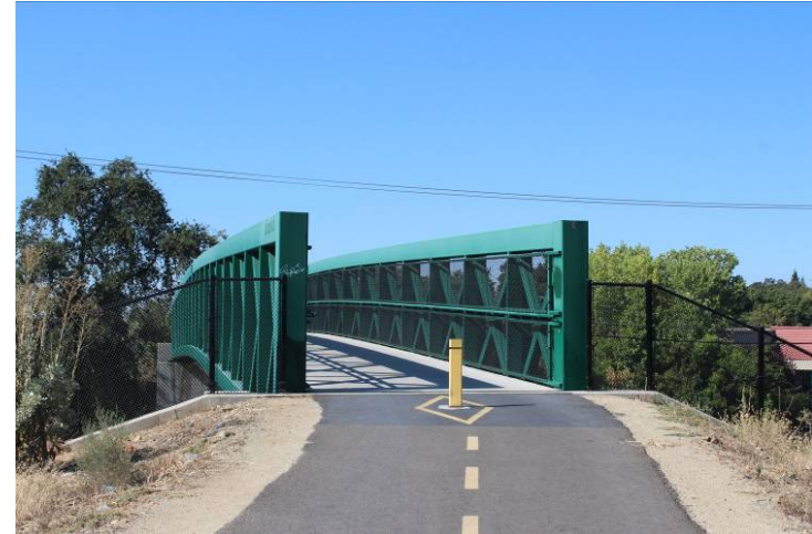
Figure 7 – Prefabricated Truss Bridge
