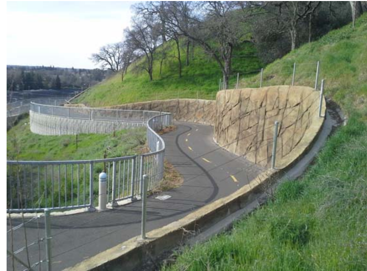
Figure 30 - Concrete Formliner Retaining Wall
